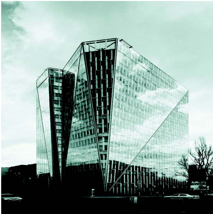
Fig. no.4 Adrian Spirescu, Crystal Tower, 2011, Bucharest http://www.adrianspirescu.ro/proiecte/crystal_tower/img/display/bo1.jpg
